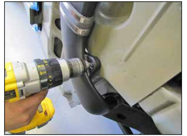
56. Using the mounting hole in the corner tube as a guide, drill a 5/64" id hole into the inner body panel.
