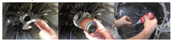
2) Install the small spacer for the plastic pipe behind the mounting tab. Use thread locking compound on the supplied longer mounting bolt and torque it to 18Nm.
