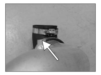
g. The opening of the coupler should be facing the same direction as the short nipple for proper alignment.
